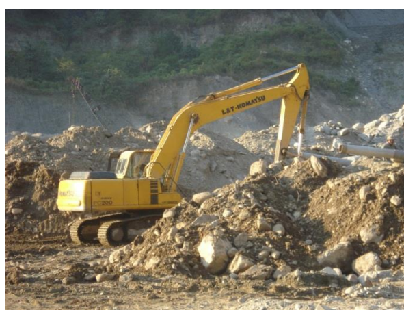
J: Construction of motorable road.
